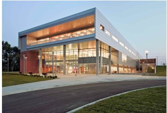
New Center for Advanced Manufacturing, Gateway Technical and Community College, Kentucky
